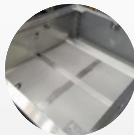
Lower sump tank normal condition
